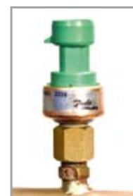
Schrader ports (for HP and LP cut-out switches)
